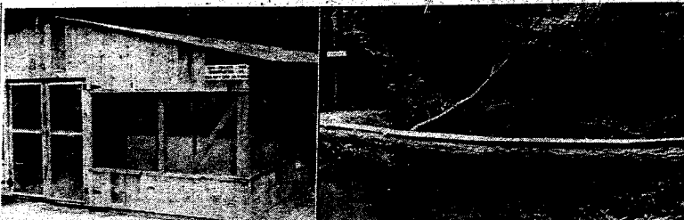
SCOUT CAMP ... A new mess hall, left, and log and plank footbridge have been constructed by units of the 577th Engineer Battalion for the Fort Benning scout camp. Company A built the mess hall, Company C the footbridge.
